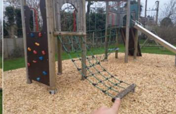
Finding: There are falls in excess of 600mm between adjacent components on the structure, in contravention of the recommendations set out in BS EN 1176 Part 1; 4.2.8.4
