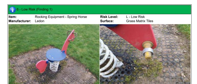
**Finding:** The end of handgrips and/or footrests have a cross **Action:** Monitor - No remedial work recommended section of less than 15cm2 and fail to meet the requirements of BS EN 1176 Part 6
