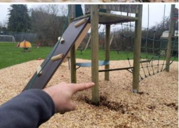
**Finding:** There are areas or parts of the timber on the structure that have rotted (client notified)
