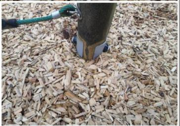
**Finding:** NOTE: Some rotten posts have been reinforced with metal legs instead of being replaced
