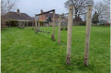
**Finding:** The inspector has some concerns about the internal condition of the timber and was unable to verify the structural integrity without further testing. We recommend a Resi-PD survey to establish the condition of the timber at it's core.
