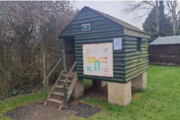
Finding: The fence forms a hard object within the falling space of the equipment and there is also insufficient surfacing provided in contravention of BS EN 1176 Part 1
