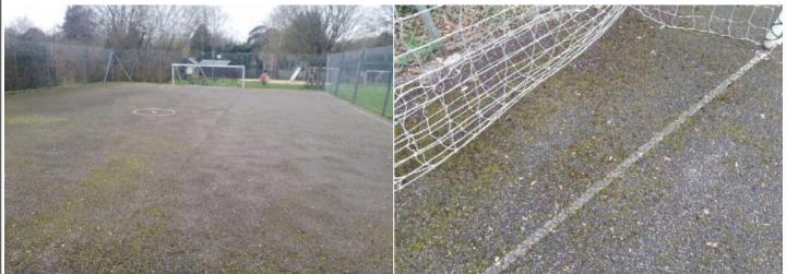
**Finding:** There is algae, silt or moss growth on the surface **Action:** Clean and treat appropriately resulting in slippery conditions
