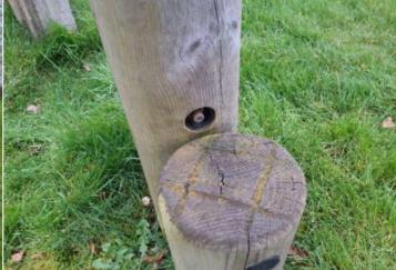
**Finding:** There is/are bolt cap covers missing or damaged on the item
